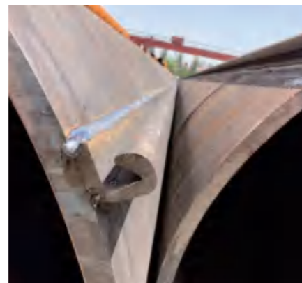
8.Clutch Lock Welding
